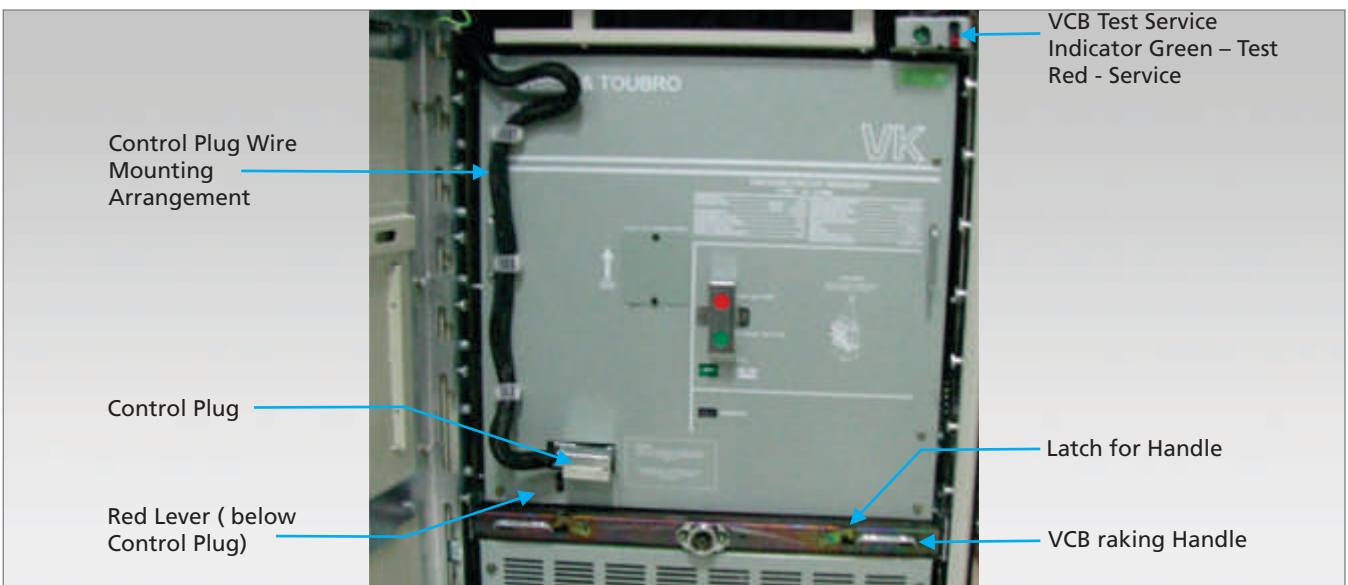
Figure 5.5 - Control Plug Arrangement
